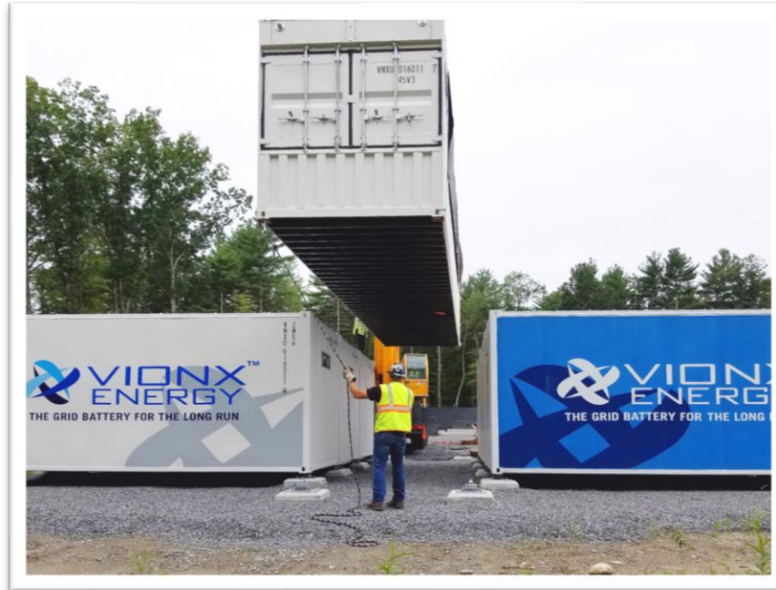
It Stacks Up: Installation of a Vionix Energy flow battery
