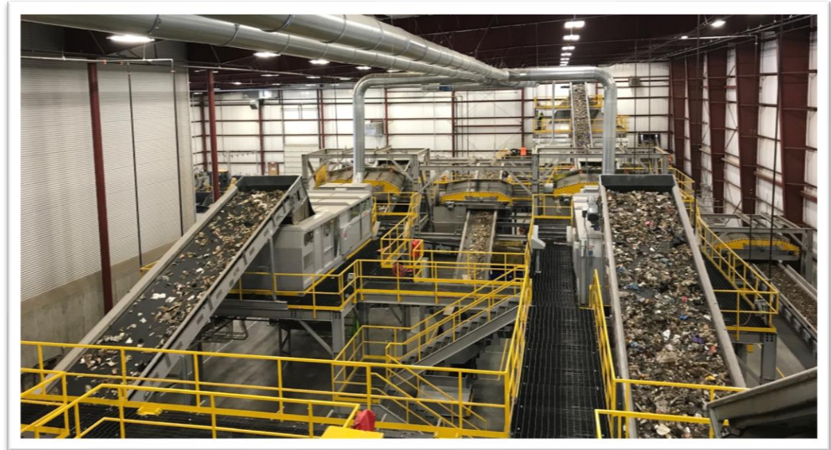
From Trash to Treasure: The Sierra BioFuels Feedstock Processing Facility
